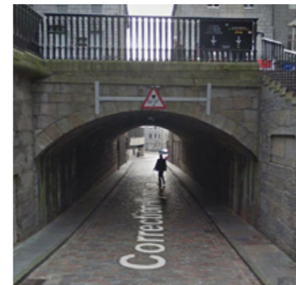
Correction Wynd underpass
