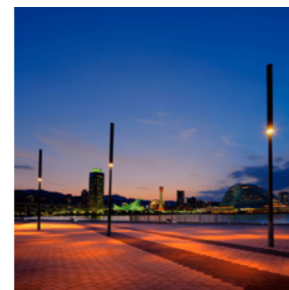
Solar powered luminaires
